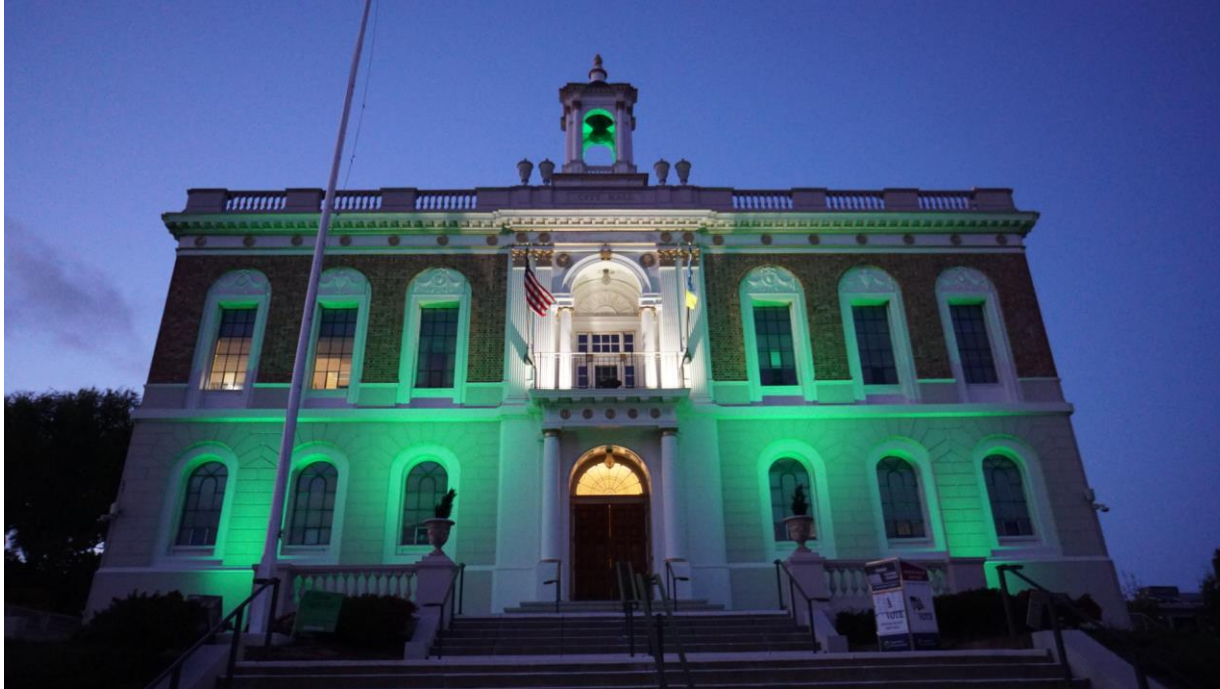
South San Francisco City Hall
